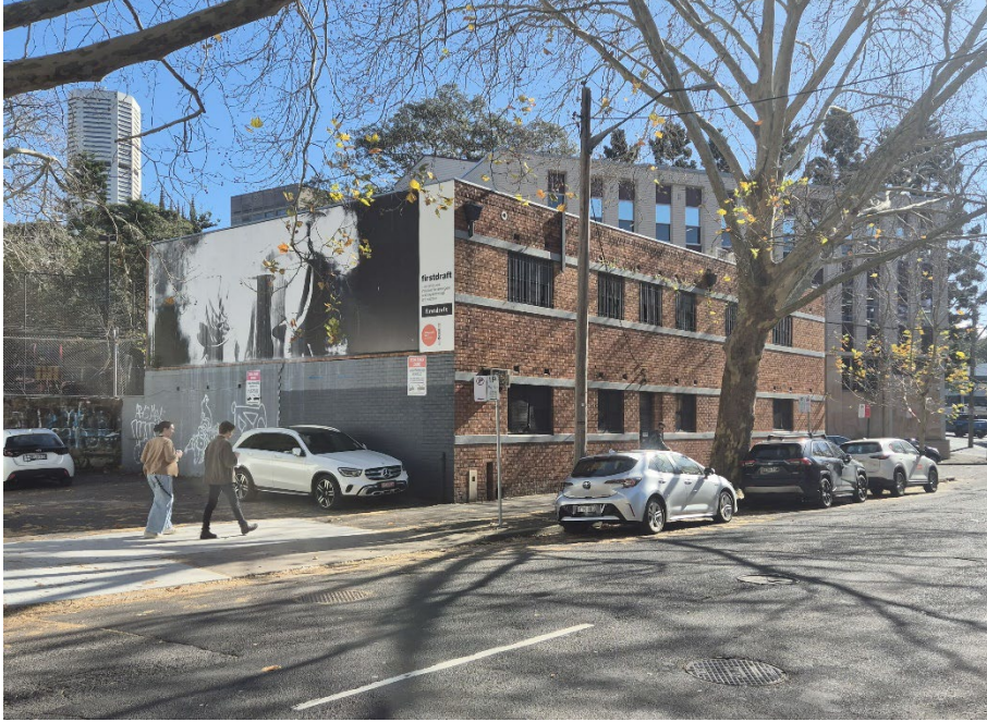
12 13-17 Riley Street viewed from the south along Riley Street.
